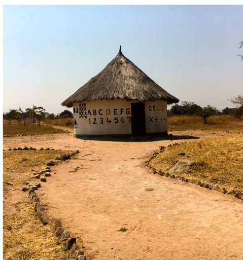
ECE classroom built using local materials in Choma District
