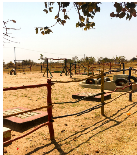
ECE play park constructed using local materials
