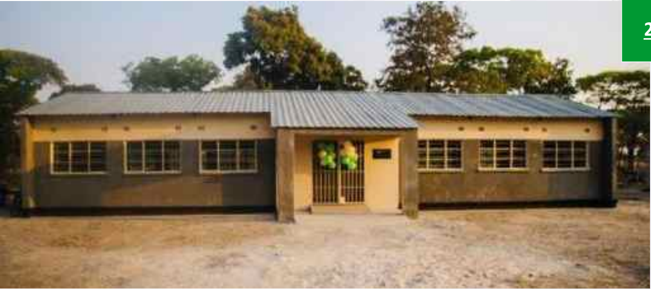
The 1X2 Classroom block built and handed over at Shambelamina Community School in Nkeyema, thanks to Hei Verden
