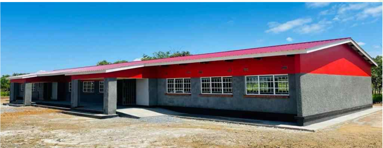
A completed 1x2 classroom block at Mwalubemba Community School in Chongwe
