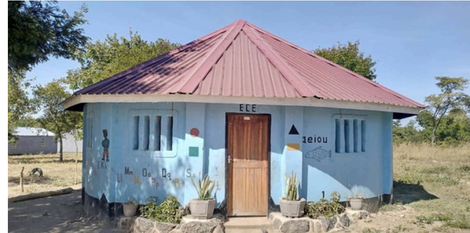
Round Huts for ECE Learning. Communities without grass, roof the huts with iron sheets
