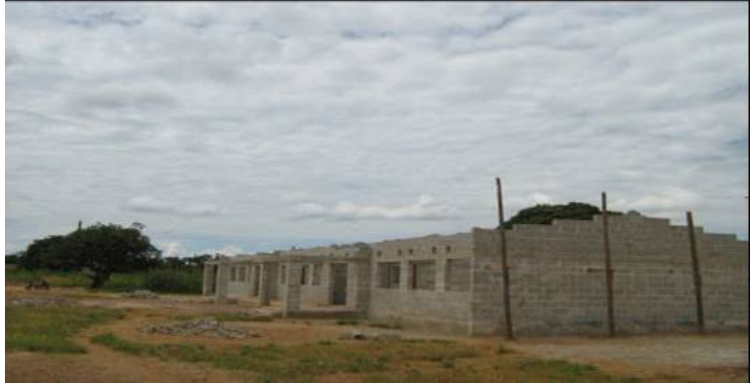
Construction of 2 x 3 classroom block at Kabwe Open Community School
