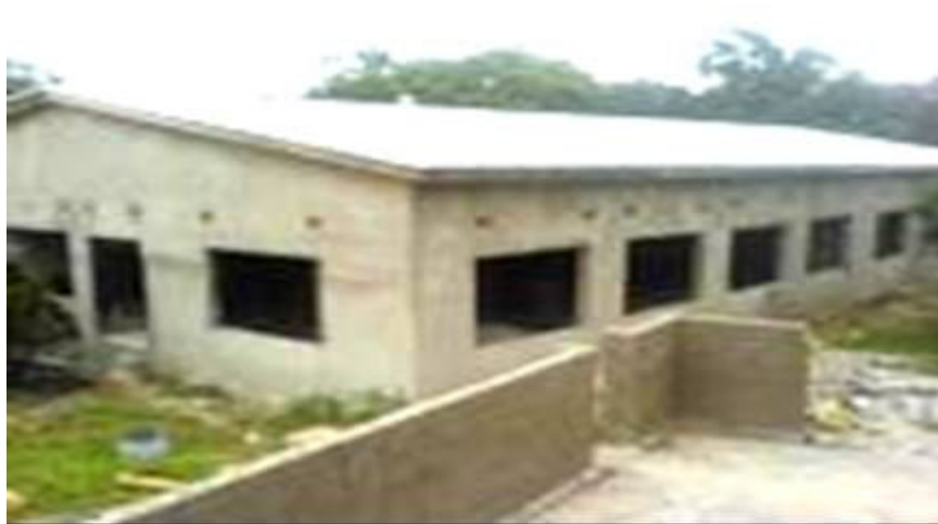
ZOCS Resource Centre under construction
